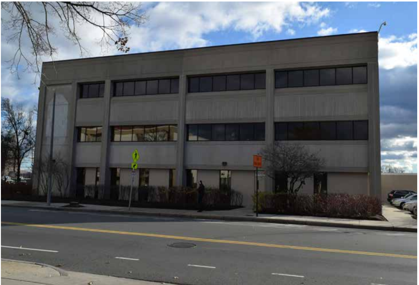
Figure 10: Existing Conditions - 114 Western Avenue North Facade
